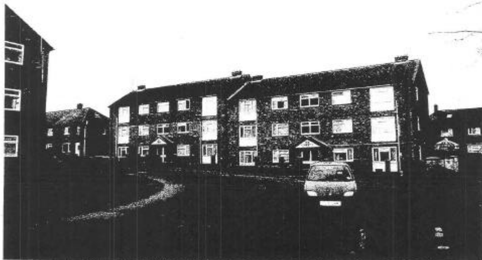
3 Storey buildings Seckwell Avenue, Franchinagh, and semi detached adjacent houses.
