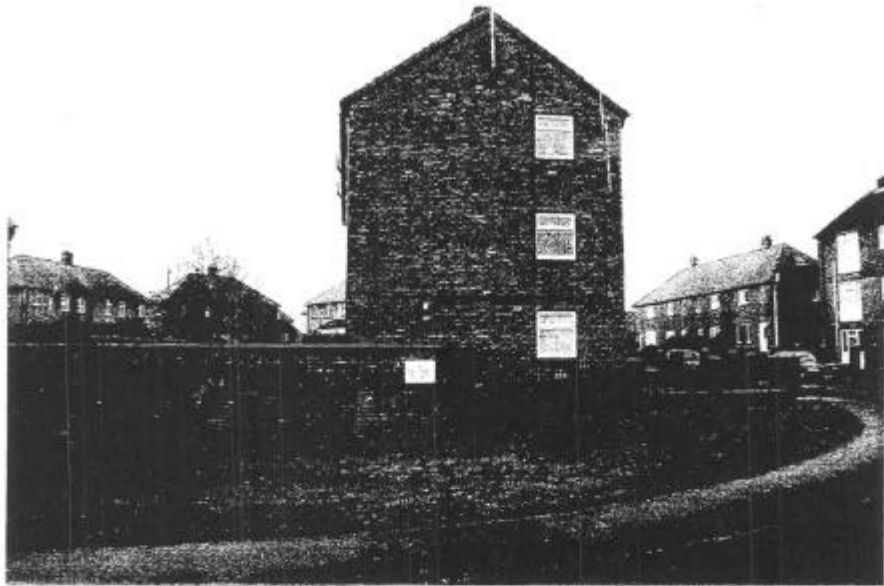
3 Storey Buildings Stockwell Avenue
